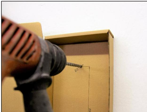
**Fig. 8c** Packaging box with drilling template
